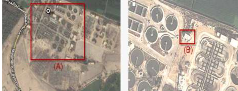
Fig. (2): A: Layout of Quhafa WWTP B: Location of Pilot Plant
