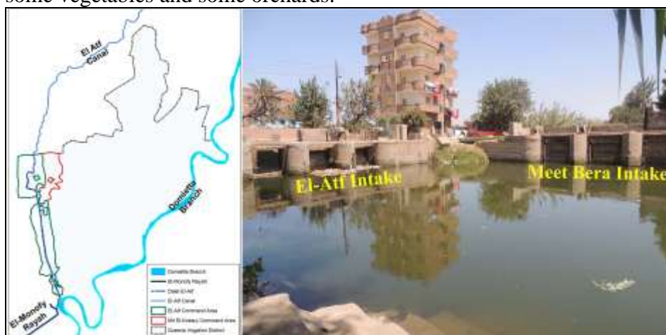
Figure (2): Schematic drawing for El-Atf canal with a photo for its head regulator
